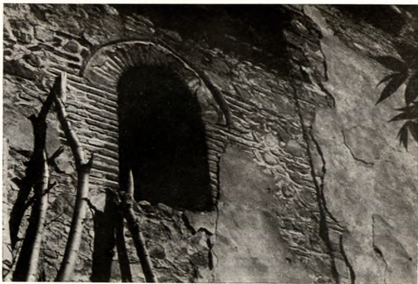
1. Serres, Mustafa Bey Mosque masonry of rear wall. Notice the seam between the two parts of the building.
